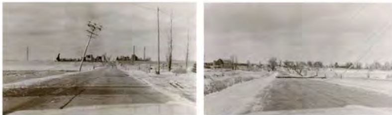
ICE STORM DAMAGE NEAR HARTFORD MARCH 4-5 1976
